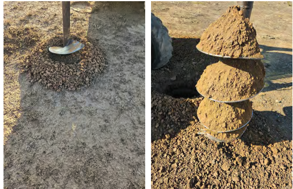
PSI being undertaken at South Coree BESS. Source: NGH
